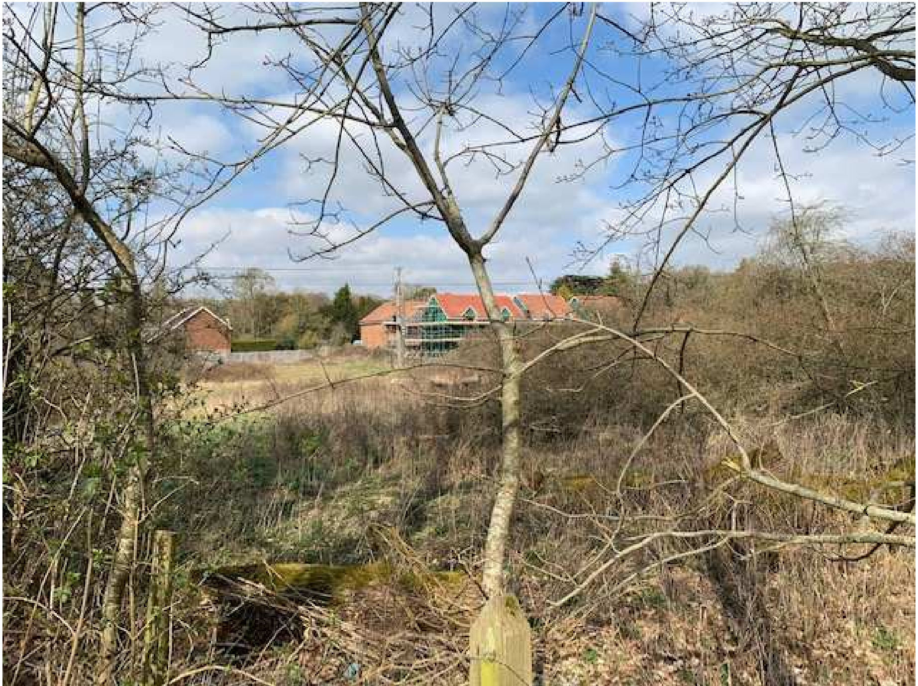
View of the application site. View looking north towards new co-op development under construction.
