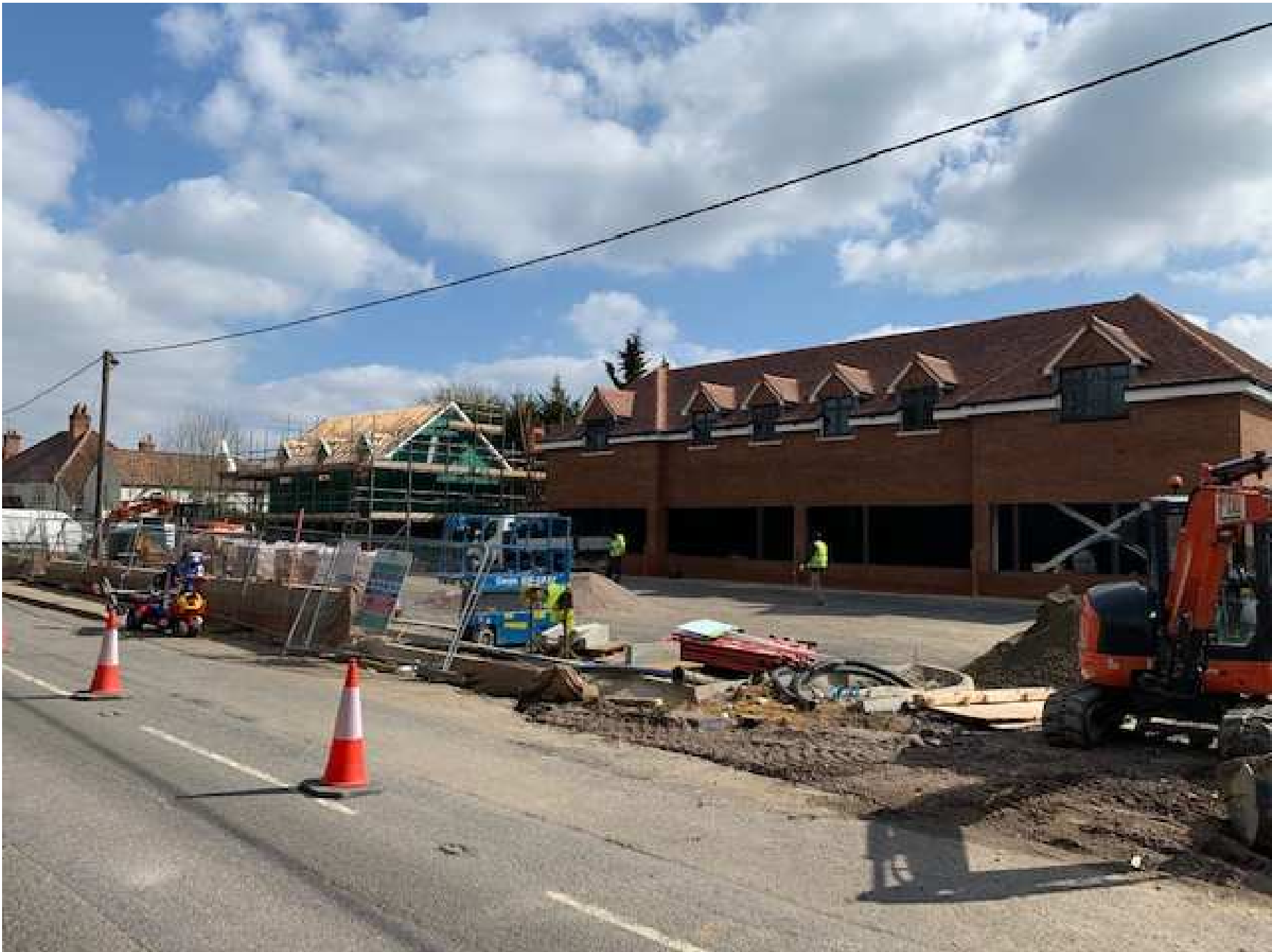
View of new co-op development under construction along Newbury Road, B4009
