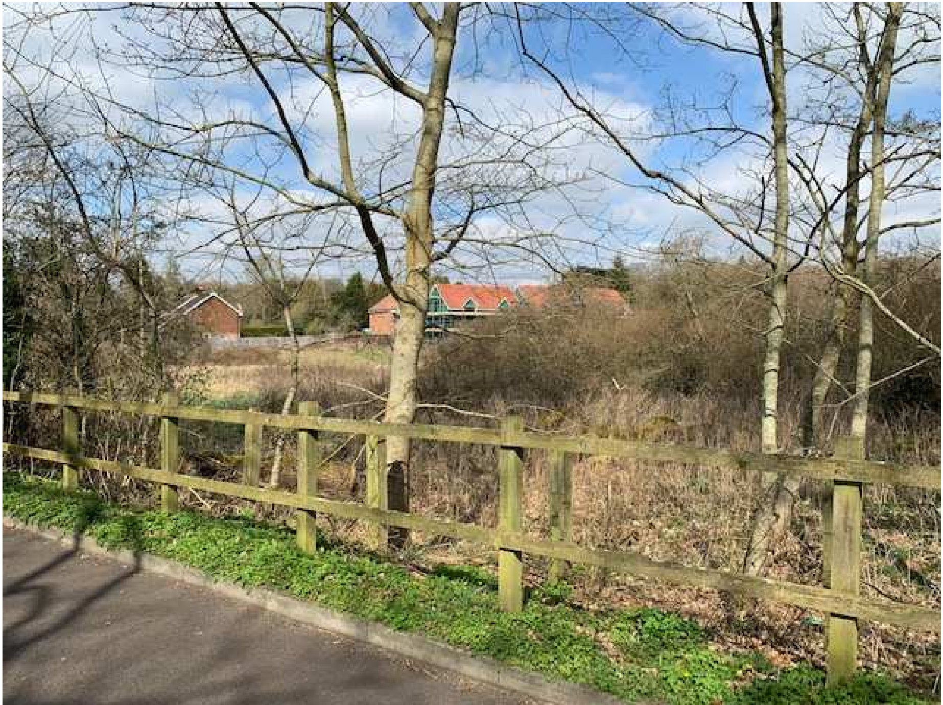
View of the application site. View looking west towards new co-op development under construction and No 2 Charlotte
