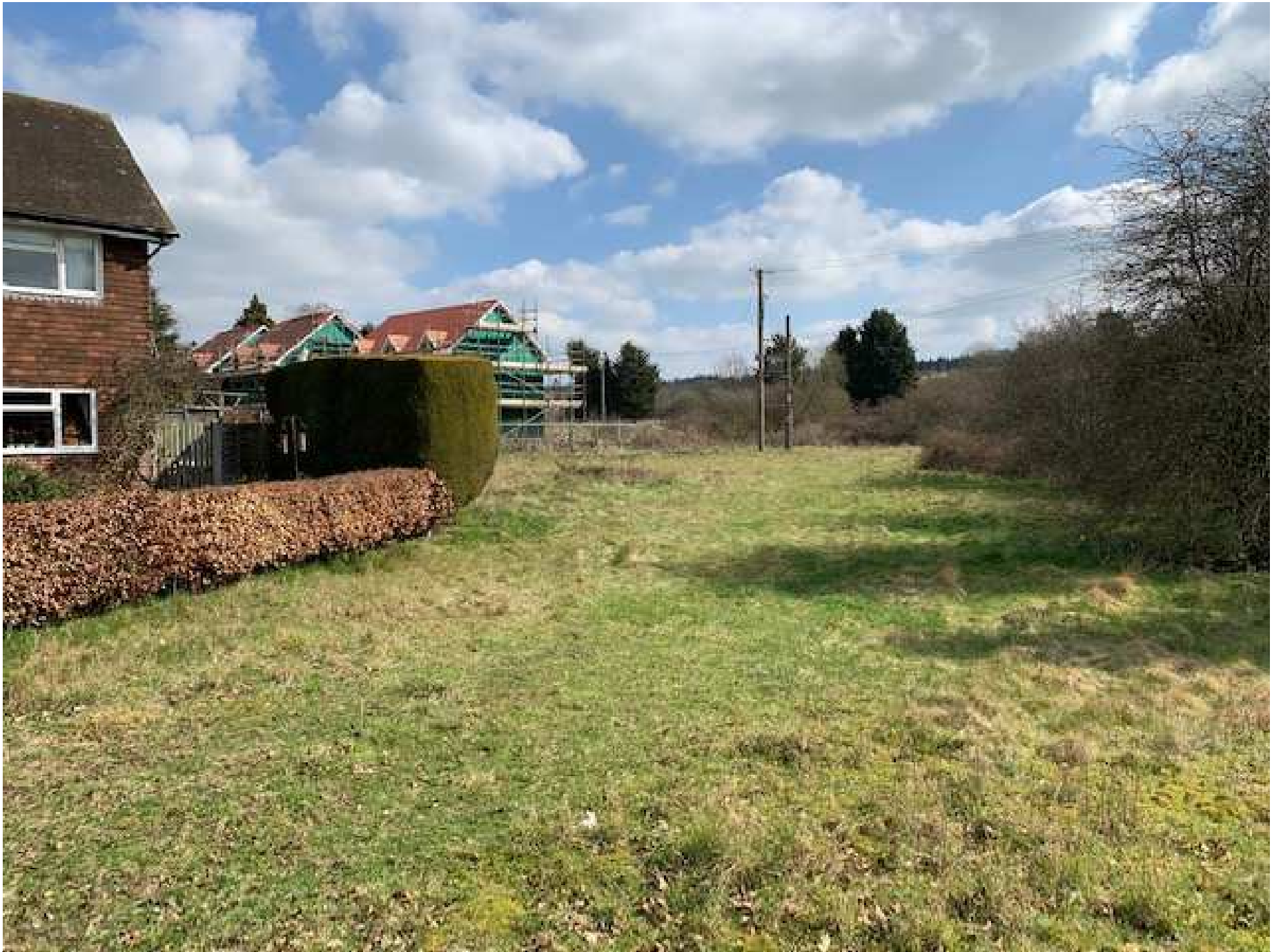
View of application site from the Charlotte Close access, showing the co-op development under construction
