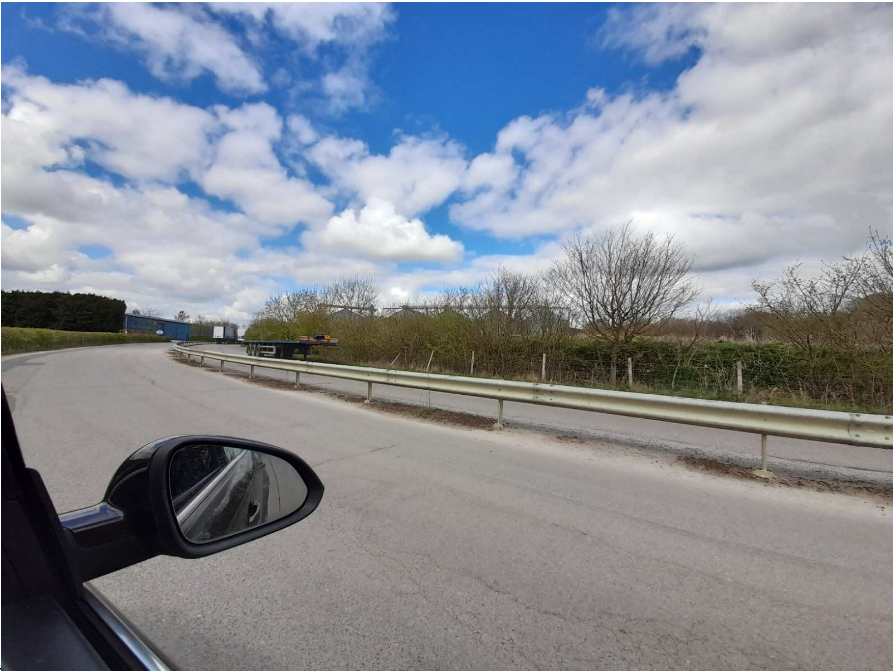
silos and industrial buildings (Looking north)
