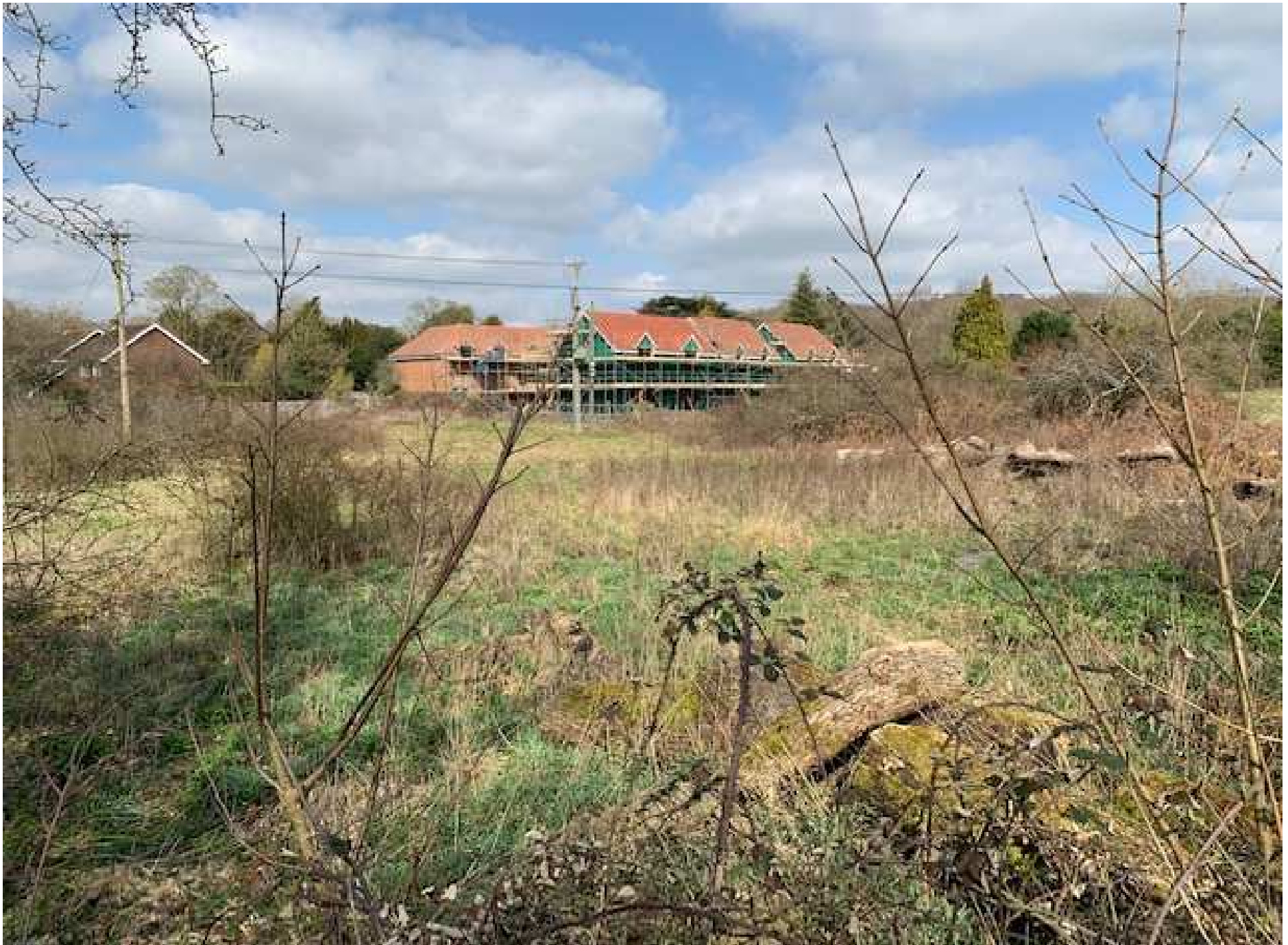
View of the application site. View looking west towards new co-op development under construction and No 2 Charlotte
