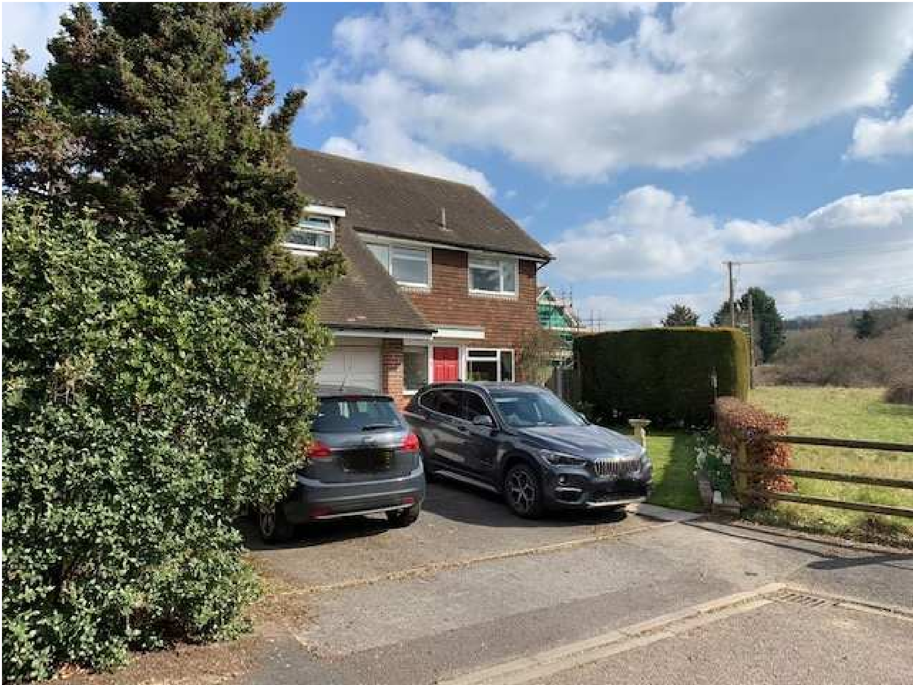
No 2 Charlotte Close – which abuts the site to the west. An example of local vernacular design
